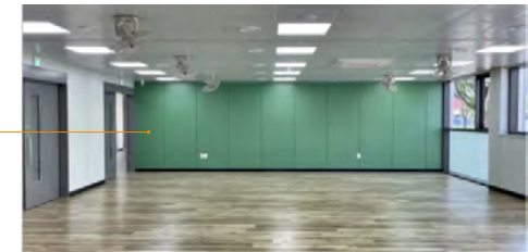
Inside a modular classroom of Banyawol Elementary School in Daegu, Korea, equipped with biomass color steel sheet
