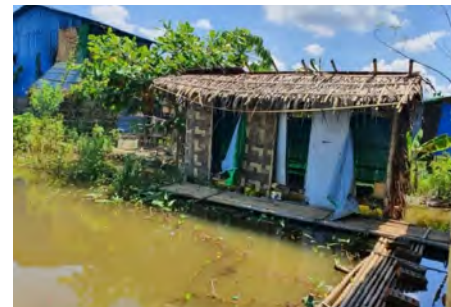
Temporary shelter huts after flood damages
