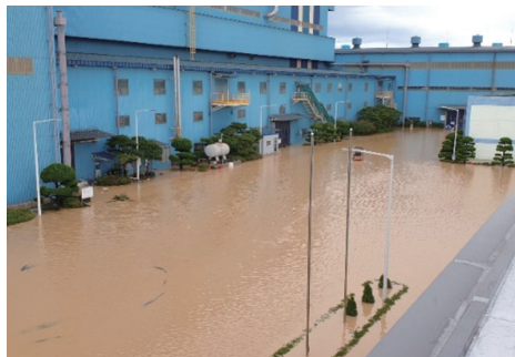
Plating factory flood damage
