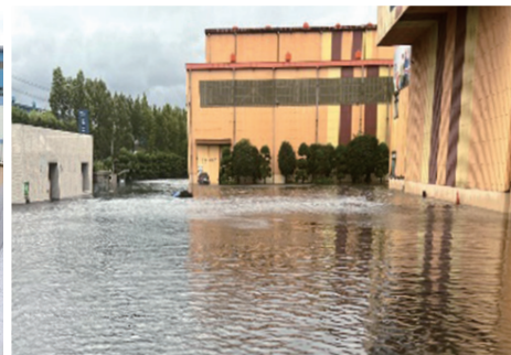
Color-coating factory flood damage
