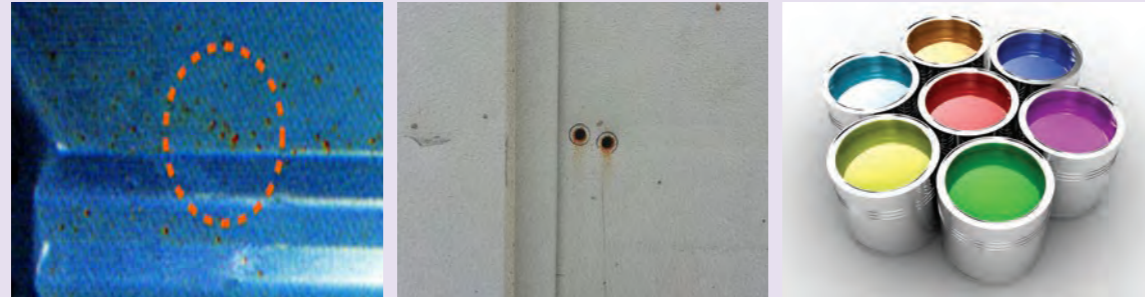
▲ Debris and inappropriate finishing
